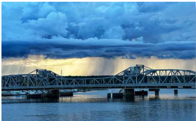
18-The Old Steel Bridge
